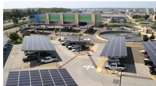
Phase 1 of the Blue Plains Solar Program included solar carport installations
