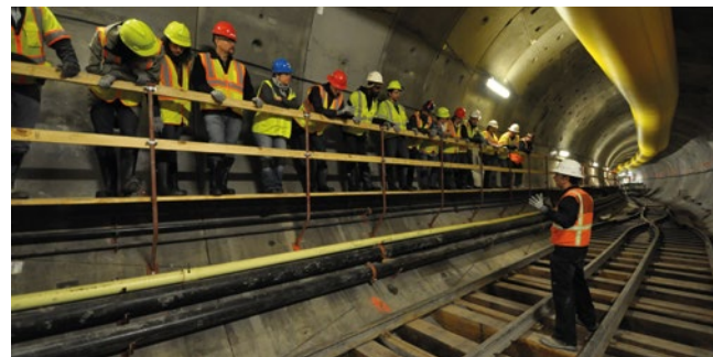
Touring the Clean Rivers tunnel construction project
