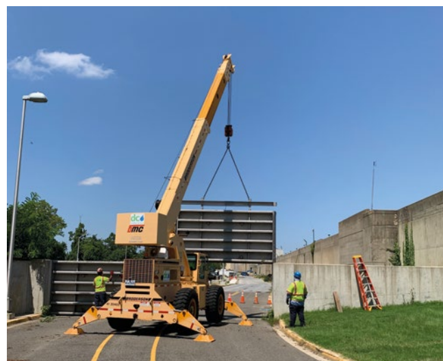
Storm gate installation at Blue Plains for flood protection
