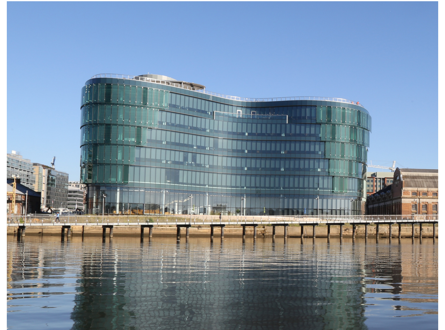
HQO, the headquarters for DC Water.
