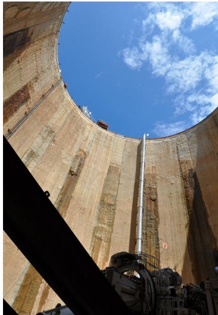
North East Boundary Tunnel boring machine in situ.
