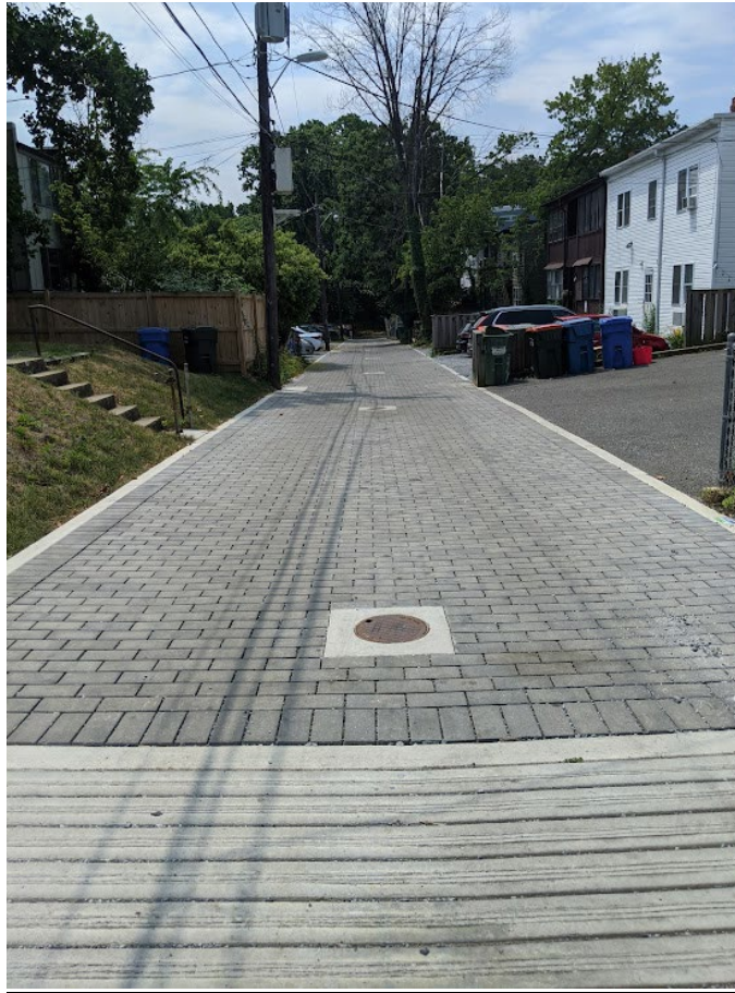
Example of concrete pad upstream of a permeable pavement facility.
