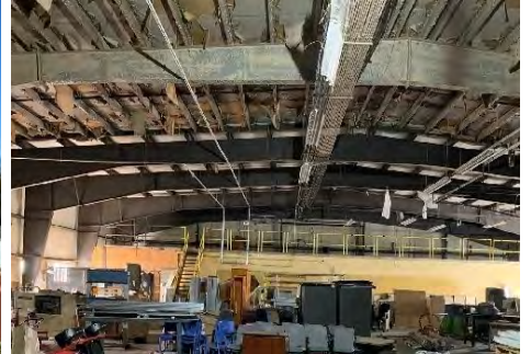
Blue Plains SB-1 Warehouse Renovation
