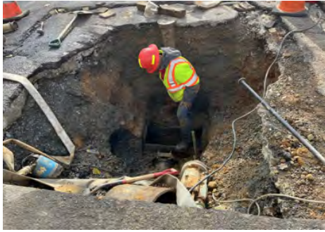
Small Diameter Water Main Rehab
