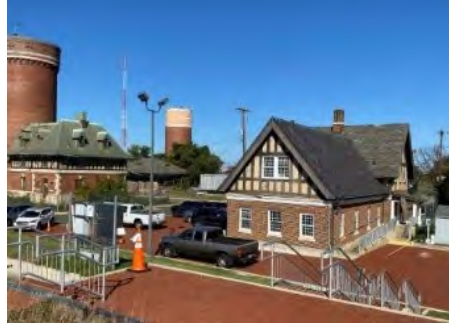
Fort Reno Renovation
