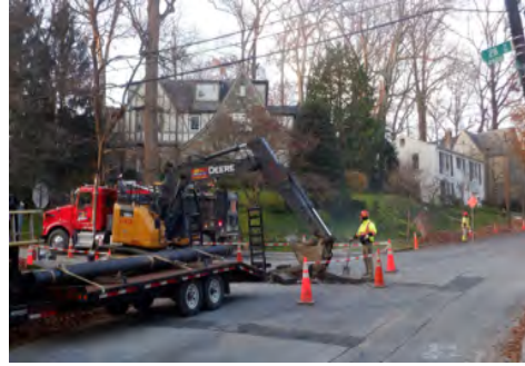
Small Diameter Water Main Rehab
