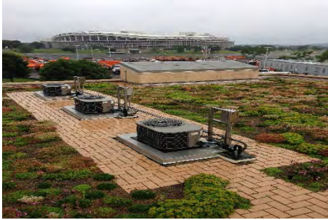
East Side Pumping Station, Green Roof
