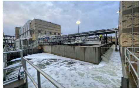
Blue Plains Clarification at Wet Weather Treatment Facility
