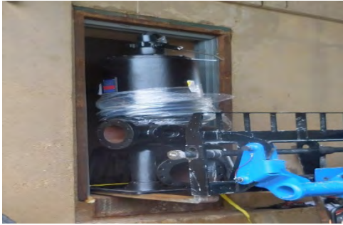
Pump Installation at Portland St Pump Station
