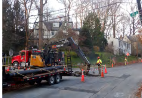
Small Diameter Water Main Rehab
