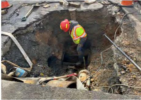
Small Diameter Water Main Rehab
