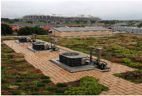
East Side Pumping Station, Green Roof
