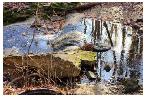
Creek Bed Sewer Inspection
