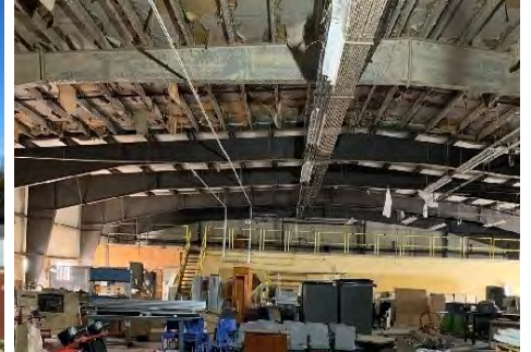
Blue Plains SB-1 Warehouse Renovation
