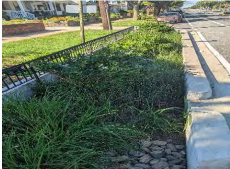
Rock Creek GI Facility
