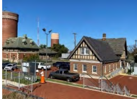
Fort Reno Renovation
