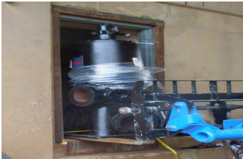
Pump Installation at Portland St Pump Station
