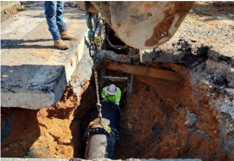
7 th St. & Constitution Ave. 20" Ductile Iron Pipe Install
