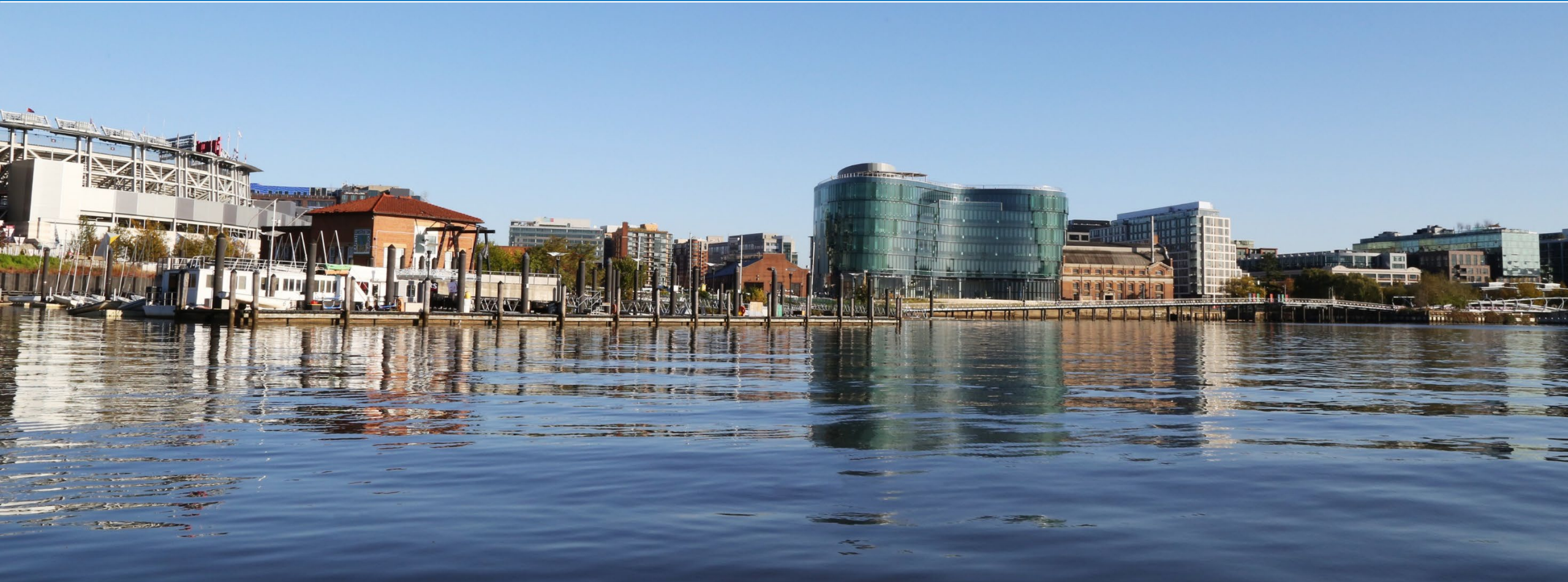
DC Water Headquarters from the Anacostia River
