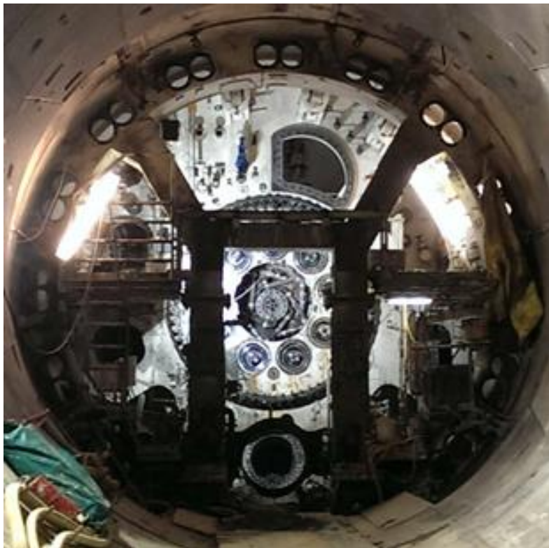
Portions of the First Street Tunnel Boring Machine left in place.
