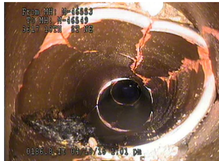
10th St at Otis St, NE (10" VCP, deformed, broken)
