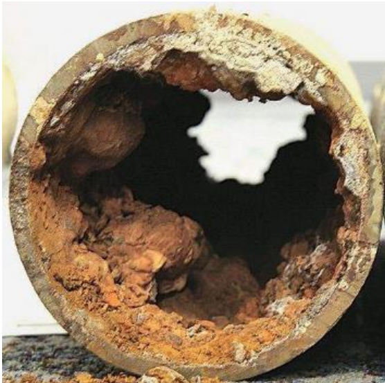
Small Diameter Water Main unlined Cast Iron pipe
