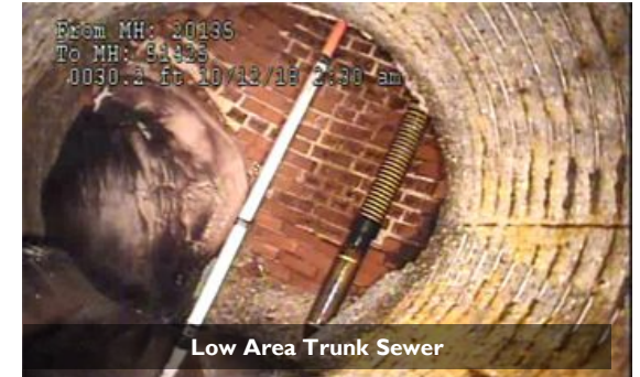
1 st and Canal Stormwater Pump Station
