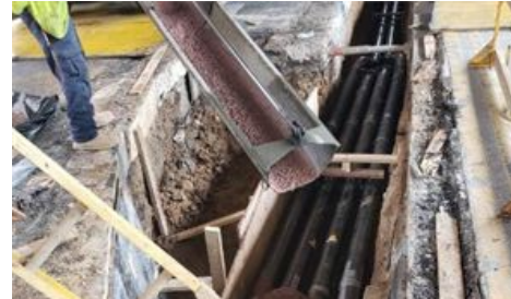
Duct Bank Work at CSO 024
