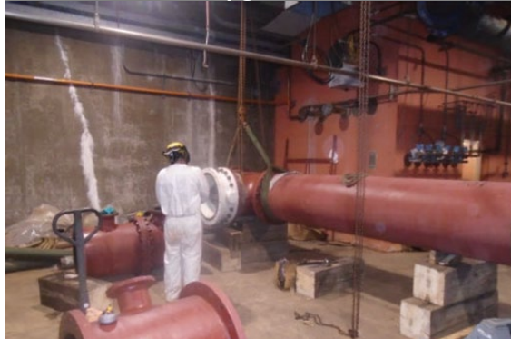
Reclaimed Final Effluent Pump Station Upgrades
