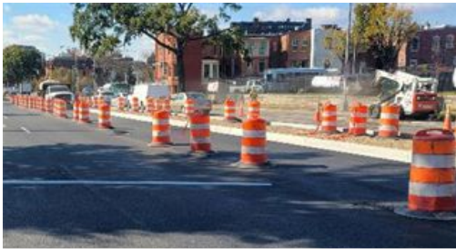
Florida Ave Restoration
