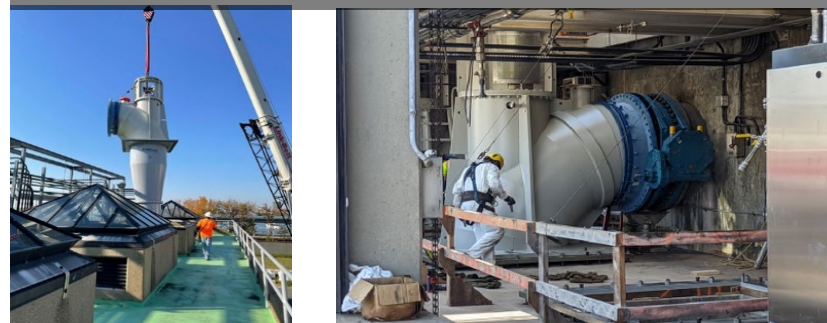
Filter Influent Pumps 1-10 Replacement Project
