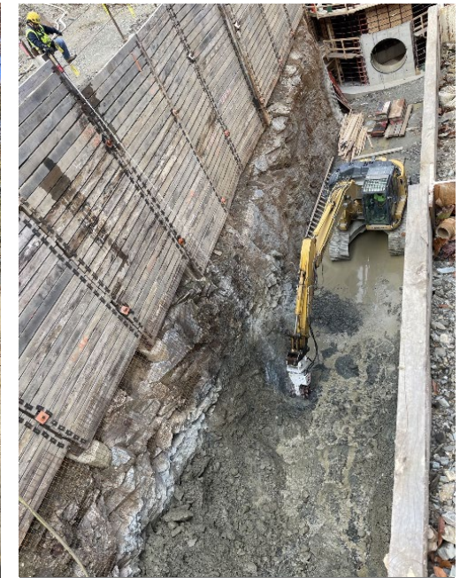
Open Trench Excavation between MH 31 and MH 30.59
