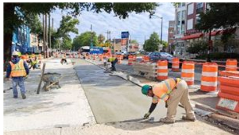
Rhode Island Ave Restoration
