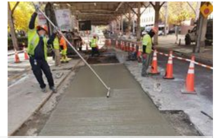
Road Restoration at CSO 024
