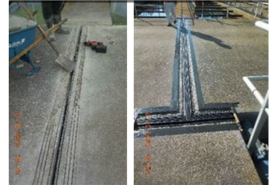
Nitrification Sedimentation Expansion Joints Repair
