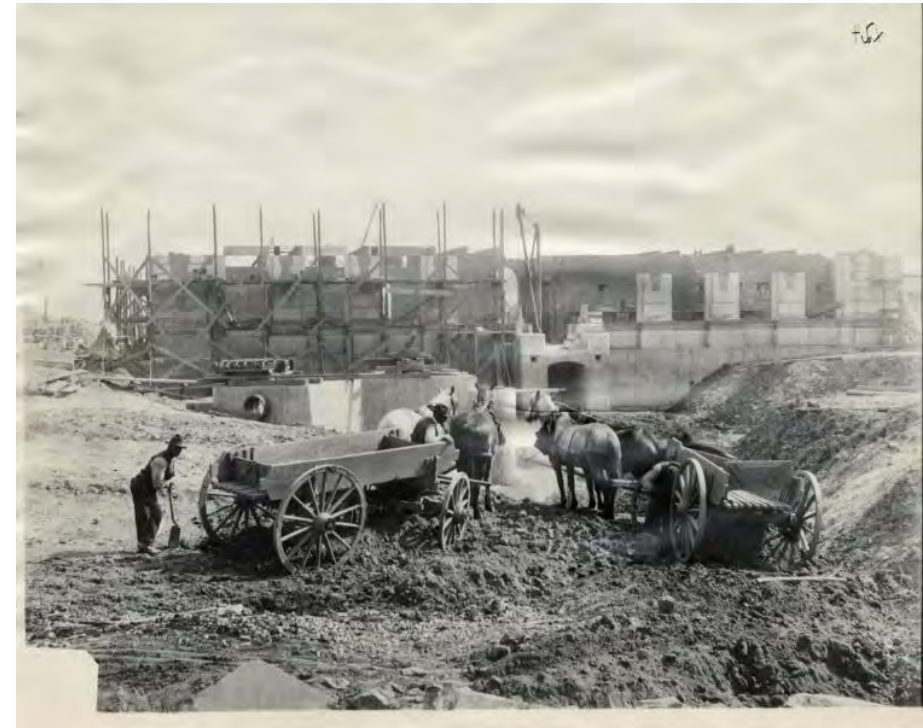
Around 1810, the first sewer structures in the District were constructed.
