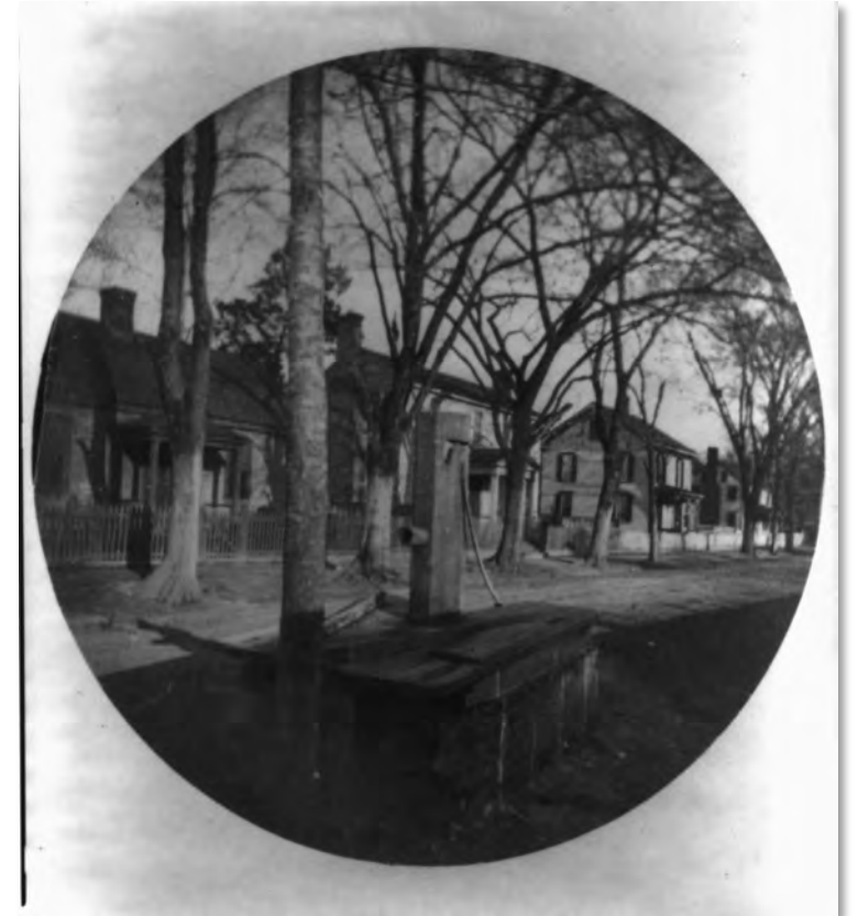
A wooden water pump on the street in Washington, DC, in 1888.
