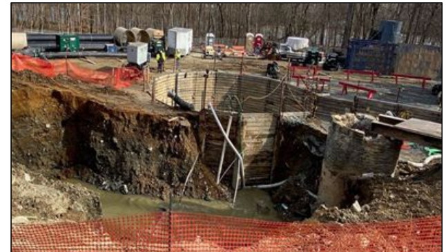
Potomac Interceptor Manhole 31
