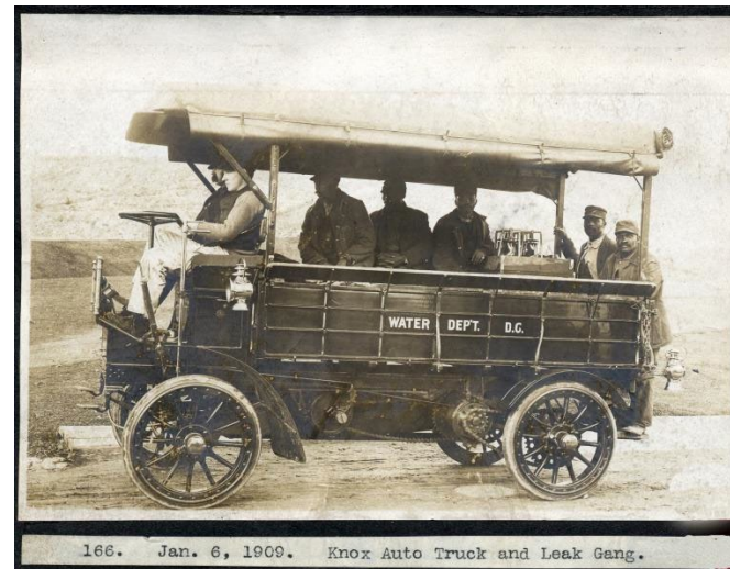
166. Jan. 6, 1909. Knox Auto Truck and Leak Gang.
