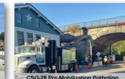
CSO-28 Pre-Mobilization Potholing
