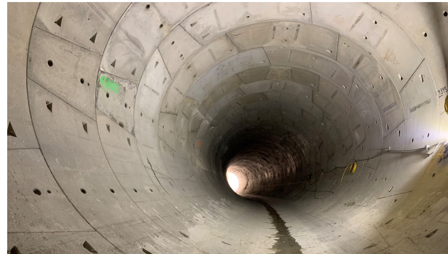
Northeast Boundary Tunnel Prior to Placing in Operation
