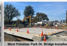
West Potomac Park Dr. Bridge Installed
