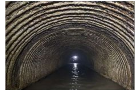
Potomac Interceptor Corrosion Resulting in Loss and Exposure of Reinforcing
