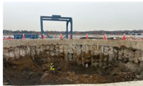
WPP- Overflow and Mining Shaft Excavation
