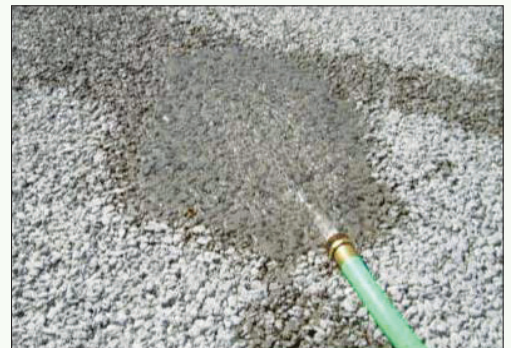
Permeable pavers allow water infiltration to prevent runoff
