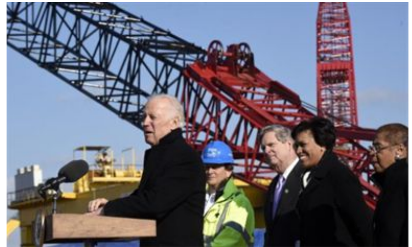
Vice President Biden Announces Infrastructure Program and Tours Anacostia River Tunnel mining site on January 16, 2015.
