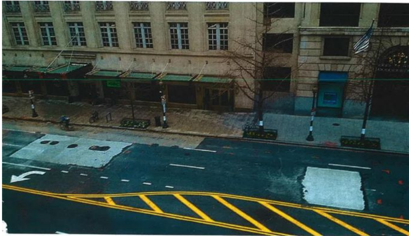
12-14-15 PCC base has cured for traffic use and edges have been tapered with asphalt for a smooth transition for vehicles.
