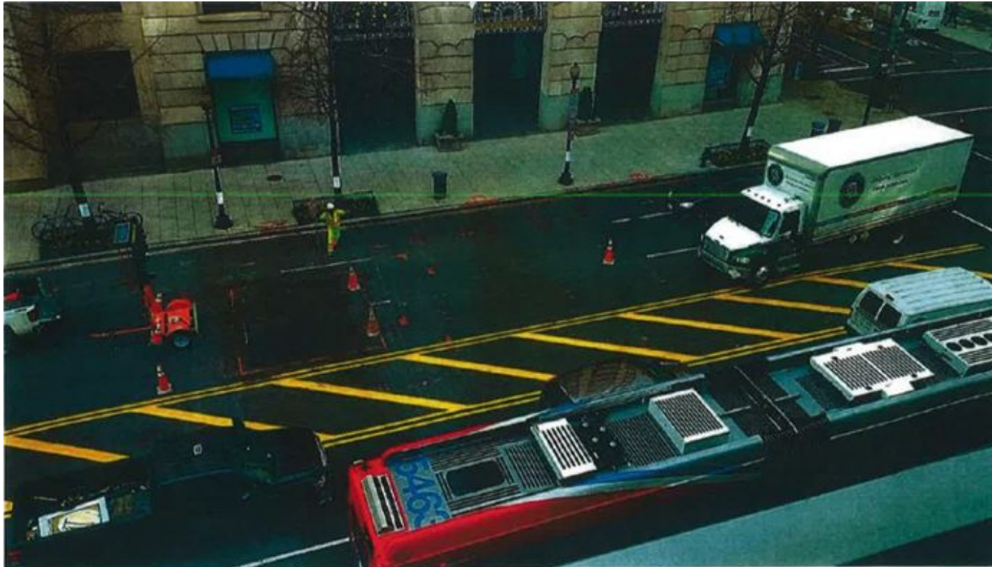
FMCC setting up additional traffic control on the North side excavation.
