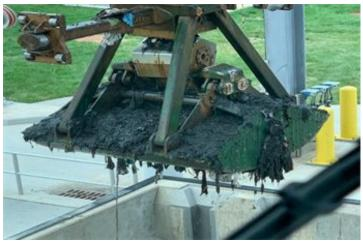
Trash, Debris and Solids Removal from Screening Shaft at Tunnel Dewatering Pumping Station
