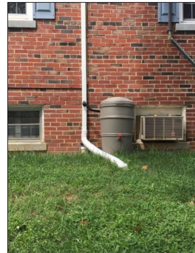
Downspout Connected to Rain Barrel
