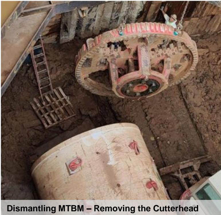
Dismantling MTBM – Removing the Cutterhead
