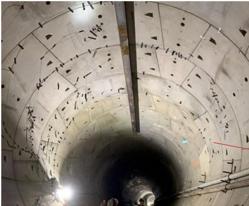
FSCT – Installed lifting beam to prep for Liner placement
