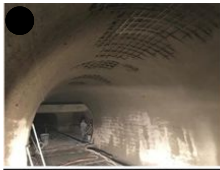
PHASE-II SHOTCRETE IN PROGRESS
