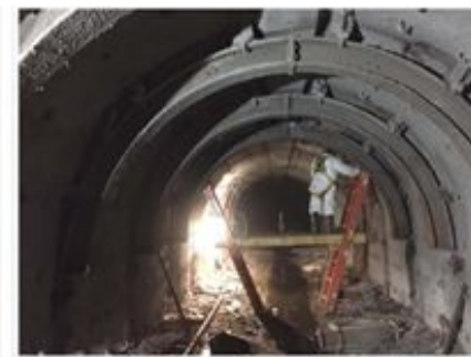
REMOVING STEEL BENTS
