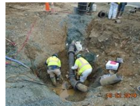
8-Inch Water Main By-Pass
