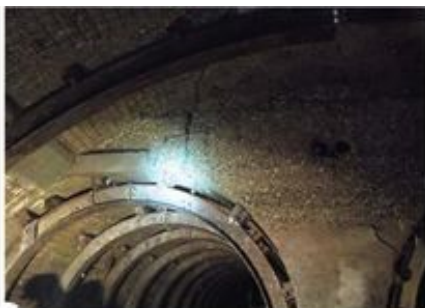
TIBER CREEK SEWER CRACKS
