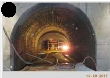
SINGLE BARREL: PHASE-II REBAR
