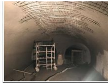
PHASE-II SHOTCRETE IN PROGRESS
