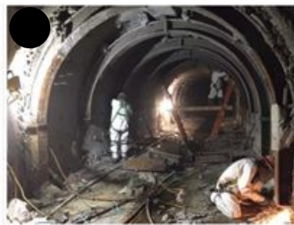
REMOVING STEEL BENTS
