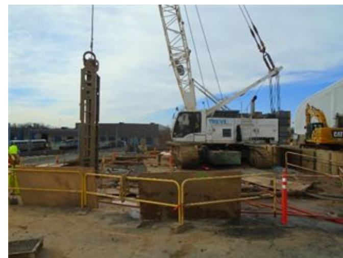
Break-In and Break-Out Panels Completed
