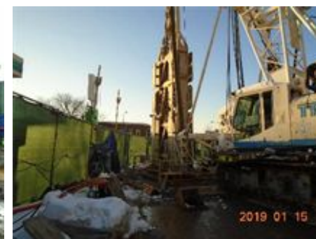
Completed Slurry Panels
