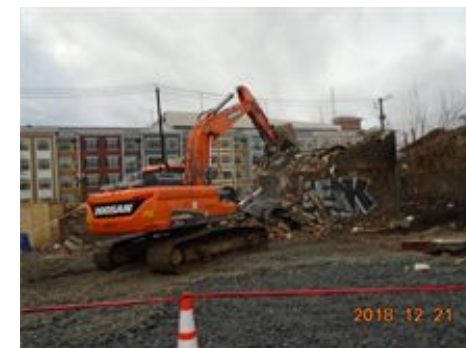
Tire Shop Building Demolished
