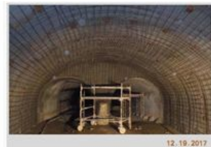
SINGLE BARREL: PHASE-II REBAR
