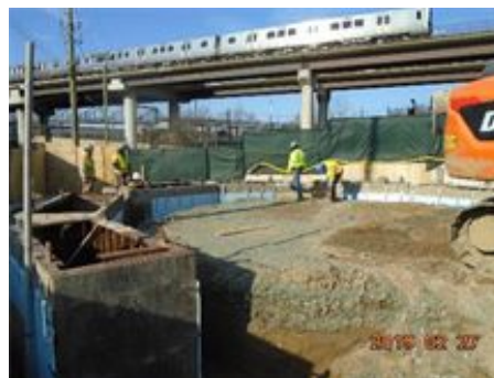
Slurry Panel Guide Wall
