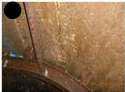
TIBER CREEK SEWER CRACKS
