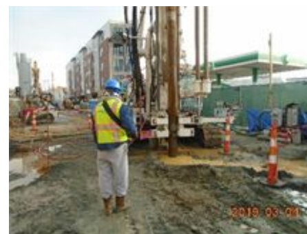
Started Jet Grout Columns
