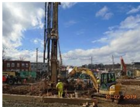
Mount Olivet Road Jet Grouting
