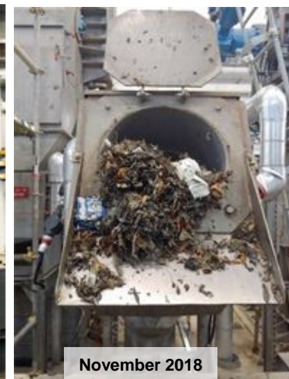
Trash and Debris Removed from CSO Captured by Tunnel at ECF Fine Screens
