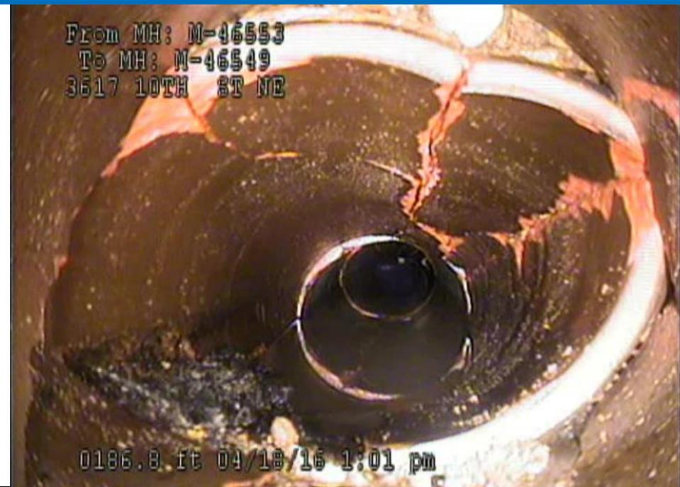
*10th St at Otis St, NE (10" VCP, deformed, broken)*
