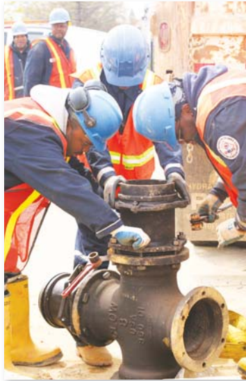
WASA crews replace an 8" water main valve in NW DC.
