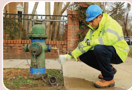
Further, sometimes hydrants are opened to blow off excess water so repairs can be made to a valve. The water pipe has to be empty in order for the repair to happen, so excess water is diverted away, usually into the street and down the storm drain.
