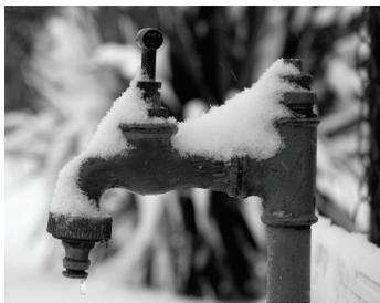
Pipes that freeze most frequently are those that are exposed to the outside and those in unheated interior areas such as kitchen cabinets, attics, garages, basements and crawl spaces.
