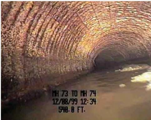
*A closed-circuit camera provides crews with an in-depth look at the condition of a sewer during an inspection.*
