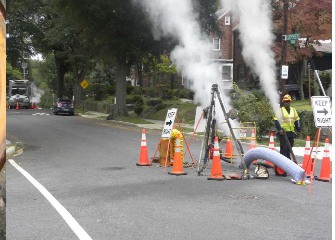
Sewer Rehabilitation - CIPP
