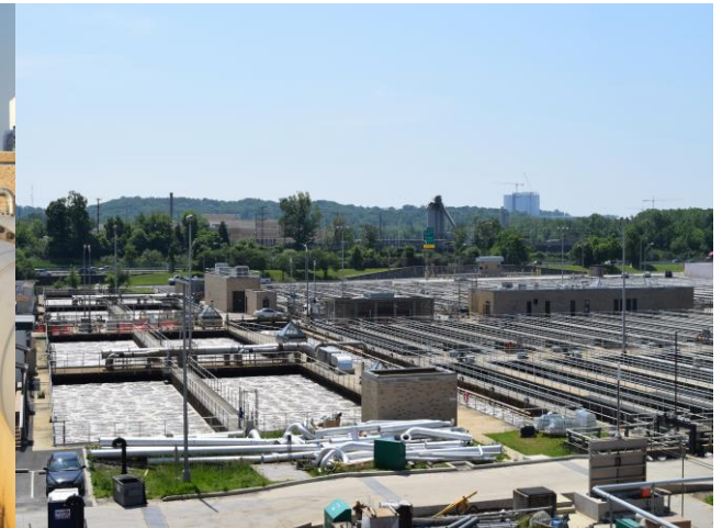
Nitrification Reactors
