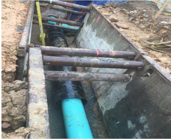
Work on Sewer Laterals
