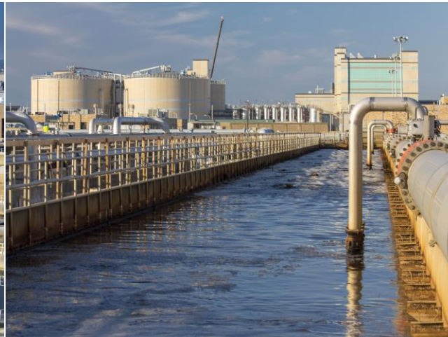
Secondary Sedimentation
