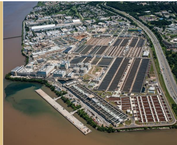
Blue Plains Advanced Wastewater Treatment Plant
