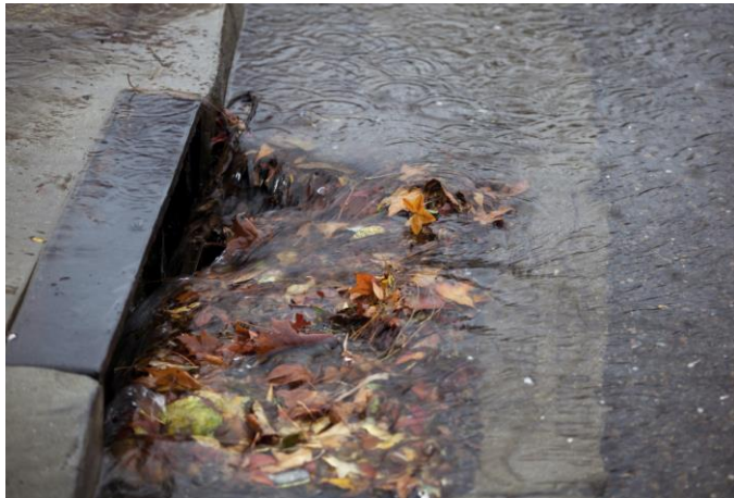
City Street Catch Basin
