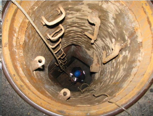
Sewer Inspection Work
