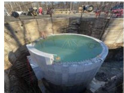
MH31 Leak Test
