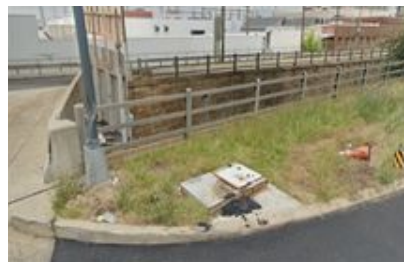
Kenilworth Pump Station entrance hatch along overpass near Benning Road.
