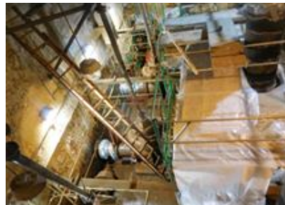
Lead paint removal ongoing at 1st & D Stormwater pump station.
