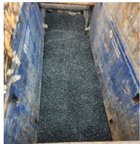
Figure 3: Temporary Repair of Collapsed Pipe
