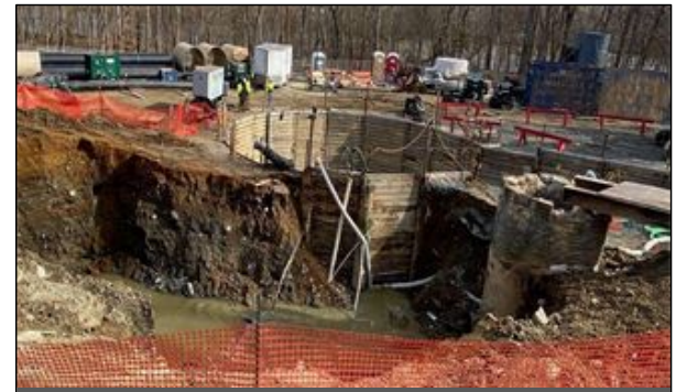
Potomac Interceptor Manhole 31
