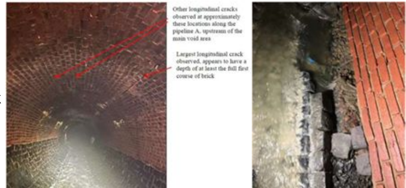
Northwest Boundary Trunk Sewer
