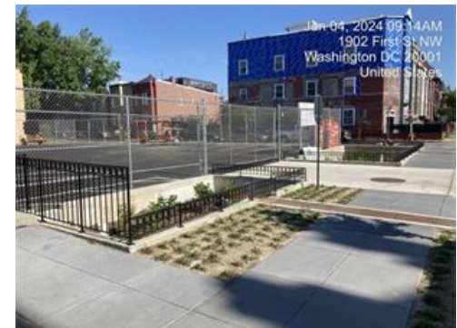
Pump Station - Site Restoration
