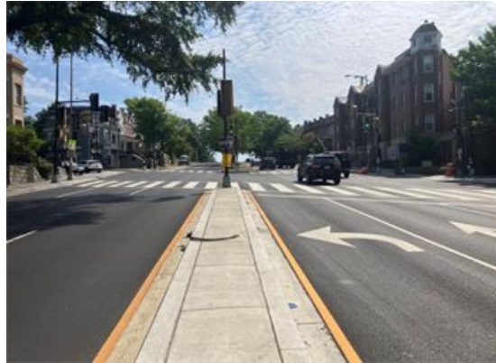
New Left Turn lane at Lincoln Road
