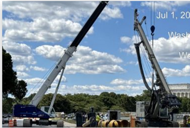
Drill Rig for Temporary Bridge Piles
