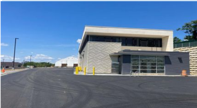
W Street - Ventilation Control Facility
