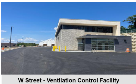
W Street - Ventilation Control Facility
