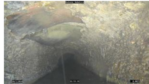
Point repair after failure
