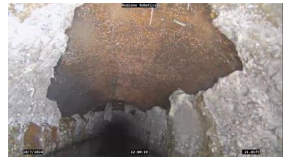
Steel pipe installed
