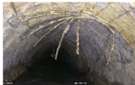
Potomac Interceptor Corrosion Resulting in Loss and Exposure of Reinforcing
