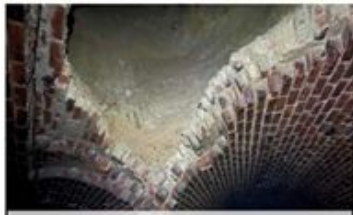
NW Boundary Trunk Sewer
