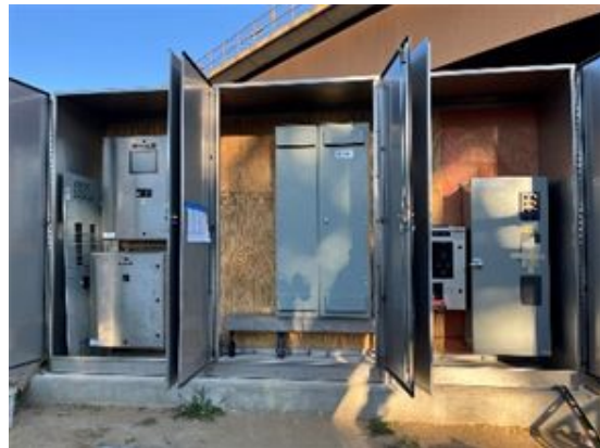
Installation of I&C and PEPCO wiring and panels.
