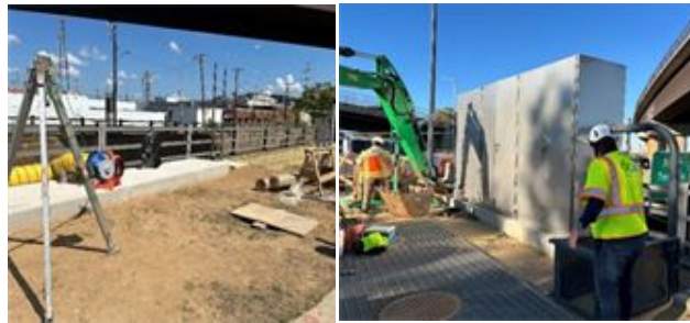
Backfilling trench & concrete slabs for cabinet support.
