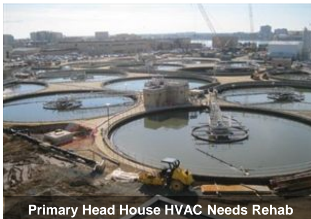
Primary Sed. Tanks Skimmer Blade Assemblies Need Replacement
