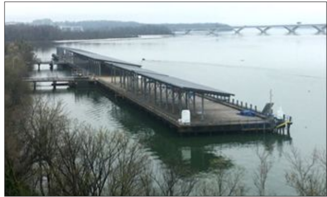
Solar Panels installed at Blue Plains dock
