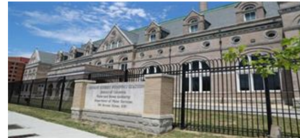
Bryant Street Pumping Station Warehouse
