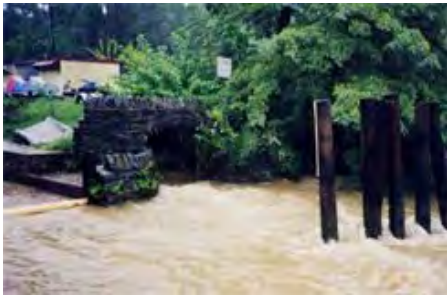
CSO Discharge to Anacostia River
