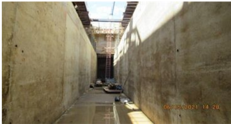
Approach Channel Walls
