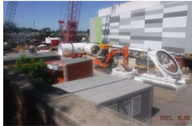
Mini-TBM Parts & Equipment on Site
