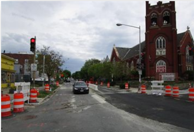
1st Street NW Road Restoration
