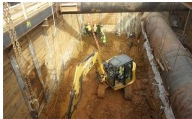
Diversion Chamber Excavation & Lagging Installation
