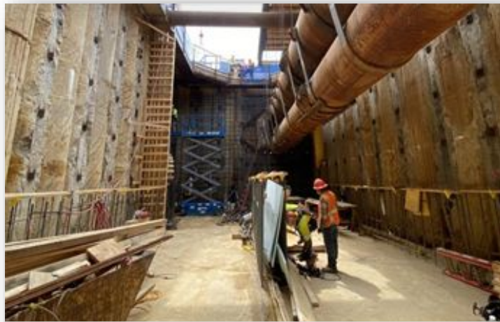
Diversion Chamber Construction
