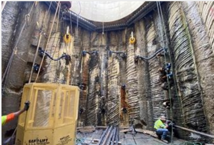
Adit Freeze Pipe Installation
