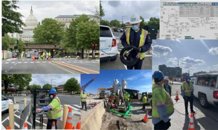
Figure 1. Staff performing above ground support in preparation of entries and connecting sensors.
