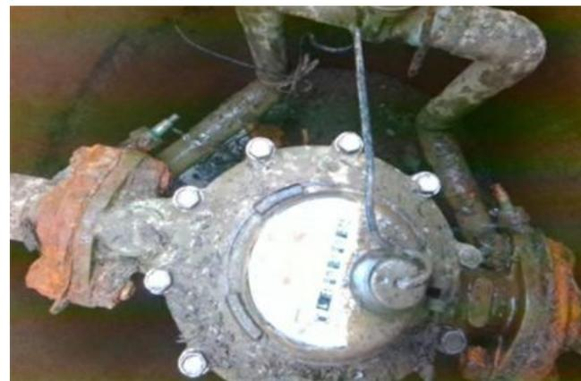
(R): Rusted and fragile flanges, both valves leaking upon arrival
