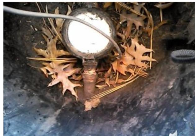
(R): Meter welded onto piping, so cannot be removed
