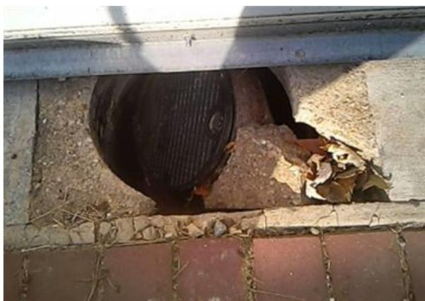
(L): Collapsed meter pit
