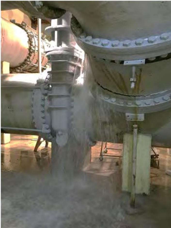
Piping segment leaking at failed flange
