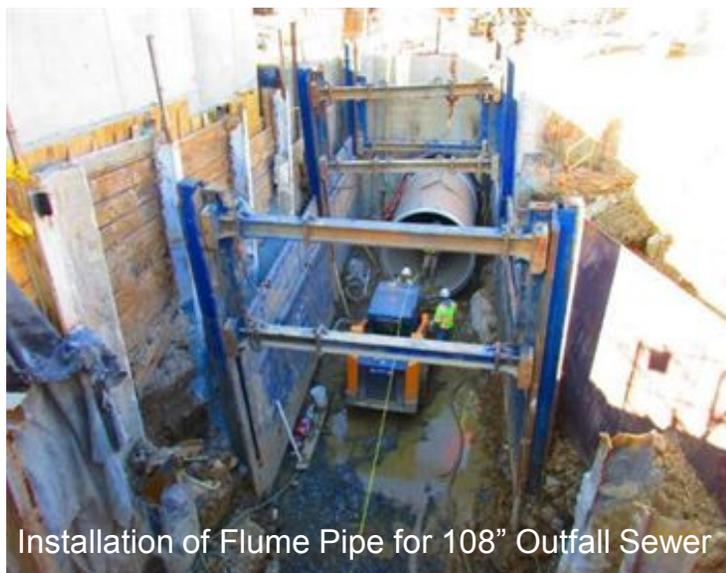
Installation of Flume Pipe for 108" Outfall Sewer
