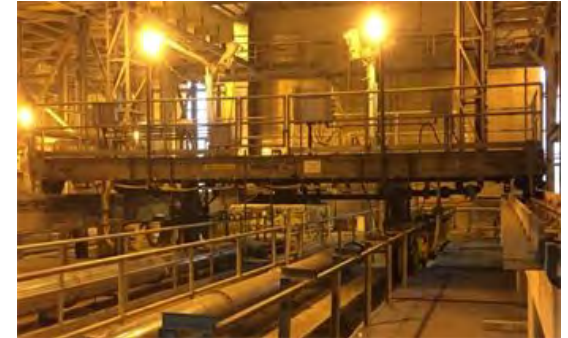
Screens, Grit & Primary Facilities Upgrades
