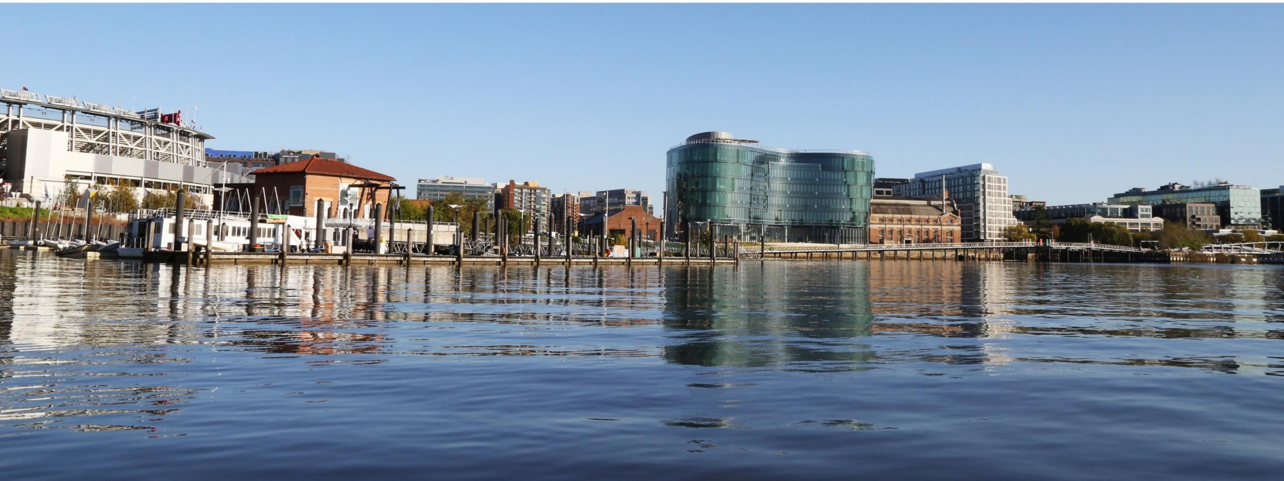
DC Water Headquarters from the Anacostia River
