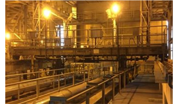
Screens, Grit & Primary Facilities Upgrades
