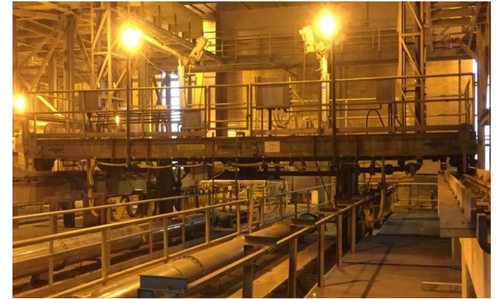
Screens, Grit & Primary Facilities Upgrades
