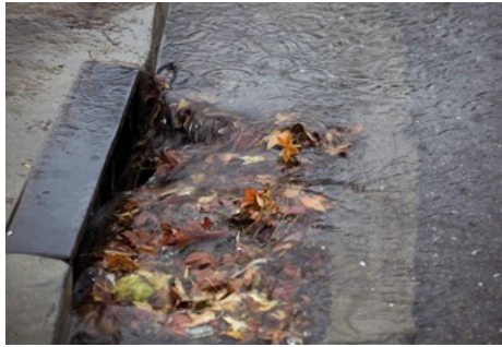
City Street Catch Basin
