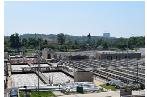
Nitrification Reactors
