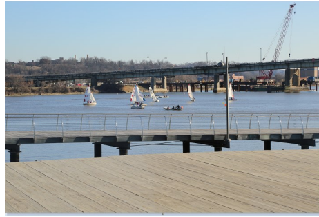
Anacostia River Tunnel Project
