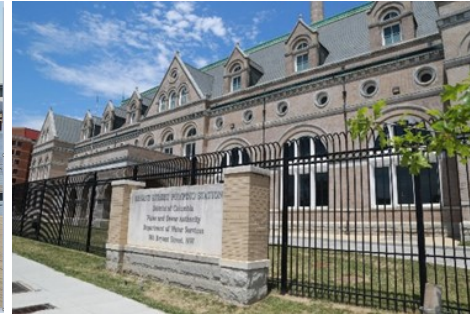
Bryant Street Pump Station
