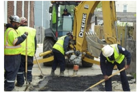
Linear Pipe Restoration
