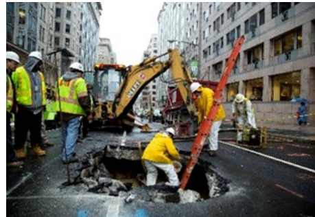
12th Street Water Main Break
