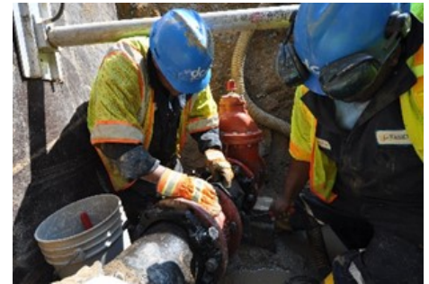
Water Meter Installation
