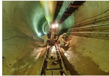
Northeast Boundary Tunnel
